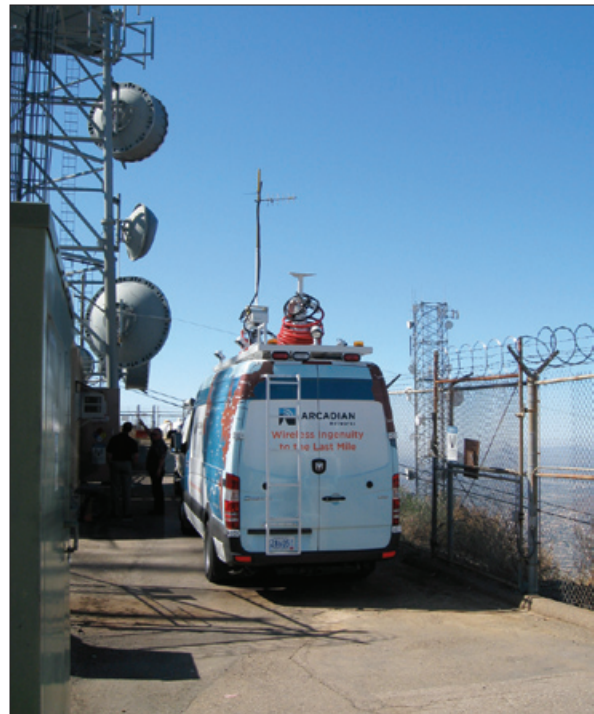
Figure 4: Arcadian field teams worked closely with Crow Wing Power crews to connect the first of 25 substations to the 700MHz network in 2007 and complete the remainder by the end of 2008.
